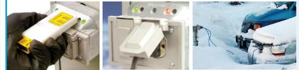
The extreme Alaskan winter makes cars so cold that many won’t start without an electrical heater that warms the engine. These heaters reduce warm-up idle emissions by 59%<sup>1</sup> (CO is reduced by almost **1 pound per start**<sup>2</sup>), but if not controlled wisely, it uses a lot of electricity.
