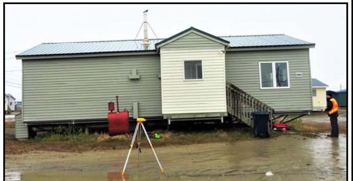
Sloping home due to thawing permafrost.
